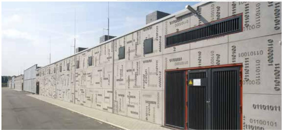
manufacture formliners with individualised textures. This is then used to manufacture the actual formliners. To help architects and engineers in their work, NOE-Schaltechnik suggests various suitable motifs for the designers to accept outright, modify or use as the starting point for their own creations.
